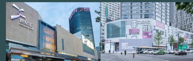
Century Link Tower
